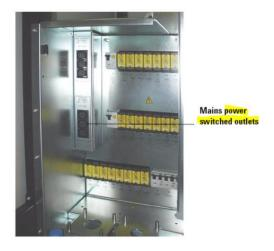
Figure 6: V93000 STH power switched outlets
