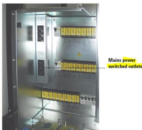
Figure 6: V93000 STH power switched outlets
